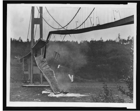
Washington, Tacoma. Suspension bridge collapses into the Tacoma Narrows. November 7. Photograph. Retrieved from the Library of Congress, www.loc.gov/item/2006687436/ , No known restrictions on publication (27.11.22)
