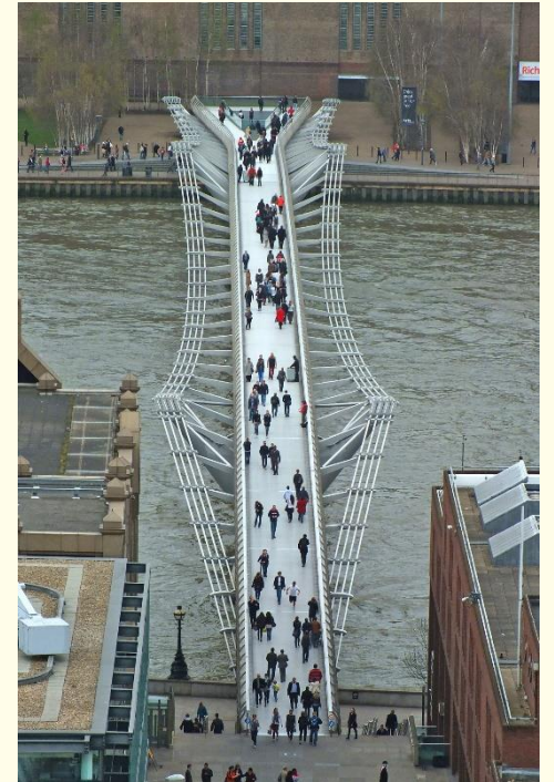
Millenium Bridge London
